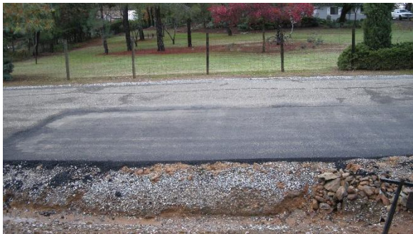
Figure 2 Calcite after Repair
